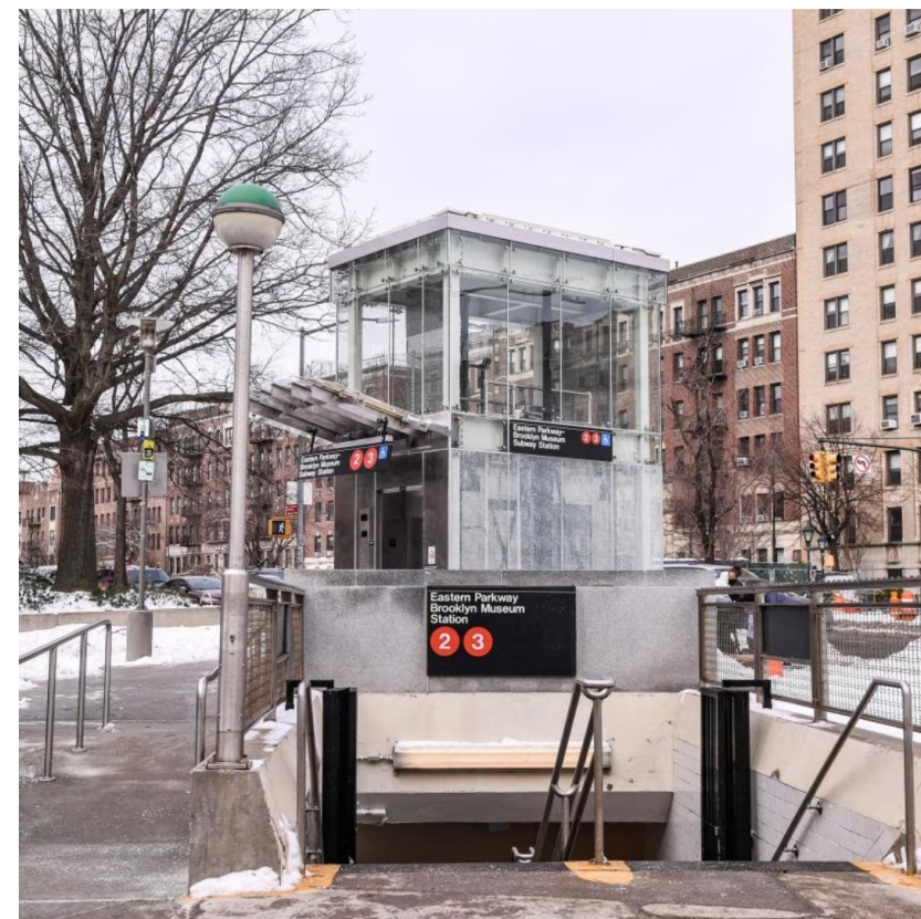
A new subway elevator installed in Brooklyn as part of MTA's campaign to make the system more accessible ( S )
